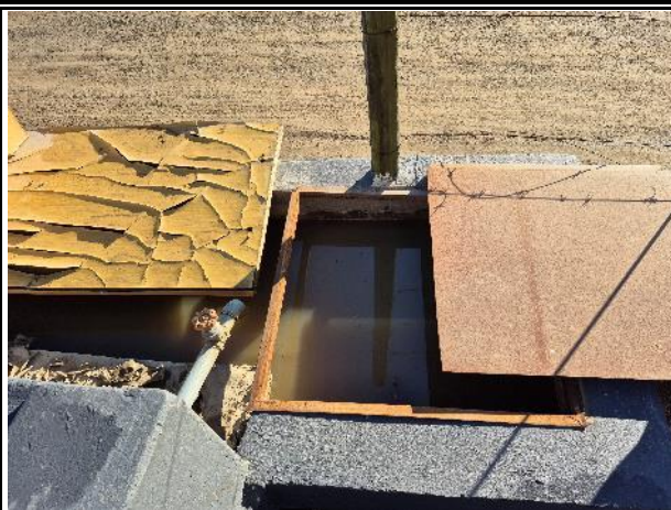
Water from the sump of diesel tank bunded area may not be used for dust suppression
