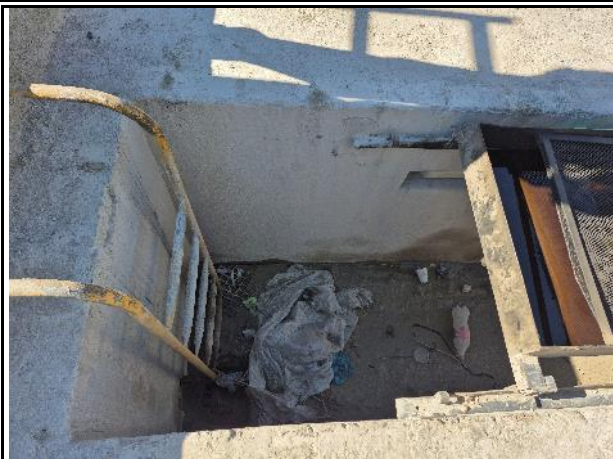
Service pit to be fitted with an oil sump
