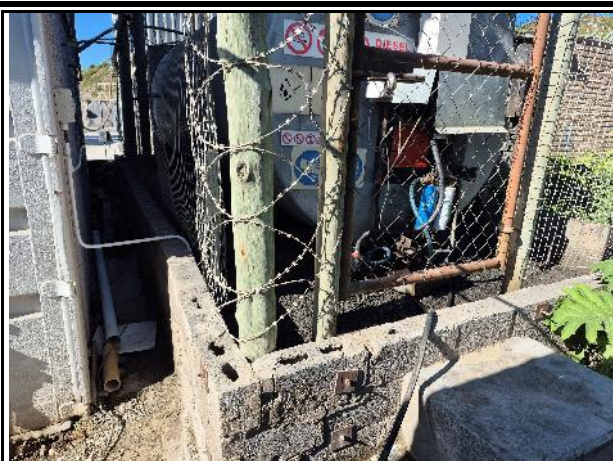
Bund of diesel tank to be sealed
