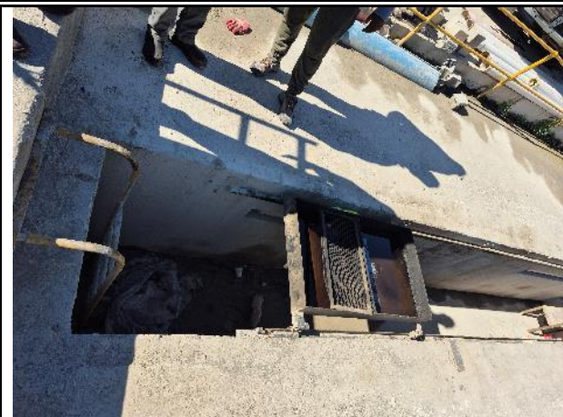
Service pit to be fitted with an oil sump
