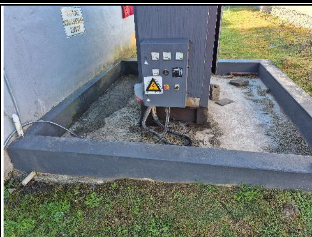
Bund of generator to be sealed
