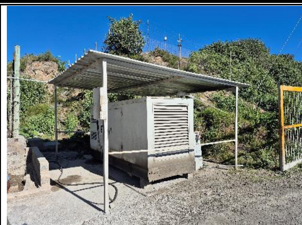
Generator to be fitted with a bund
