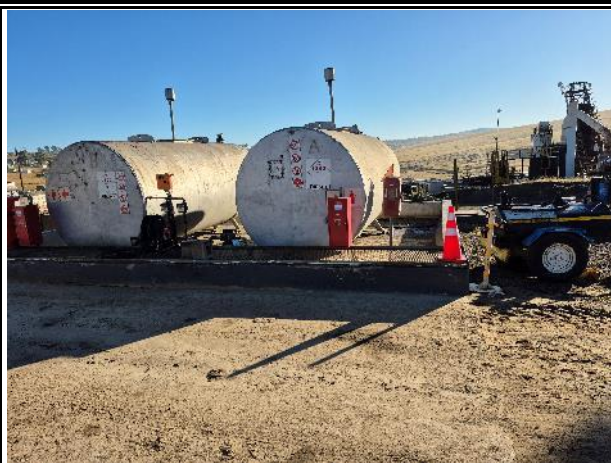
Water from the sump of diesel tank bunded area may not be used for dust suppression
