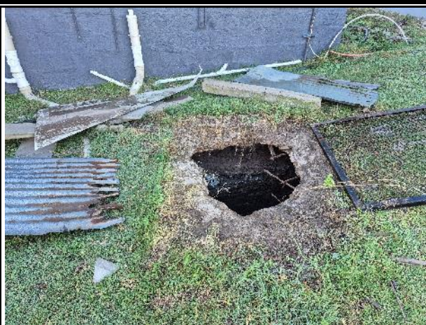
Old septic tank area being decommissioned
